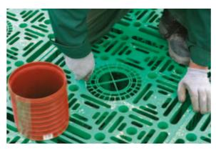
Cutting out the open-work cover of a  ${\rm d_n}$  200 mm hole located at the top of the box
