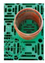
Placing a 200 mm PVC-U pipe in the opening
